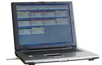
PC-SCITEQ software station overview
